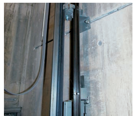
Elevator Guide Rail Connected using Cast-in Channels
