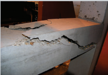
Post load test, showing ultimate shear failure mode; a continuous polystyrene strip was cast into the wall beneath the Eazistrip joint to simulate poor compaction of the concrete. The wall/slab connection remains essentially intact.
